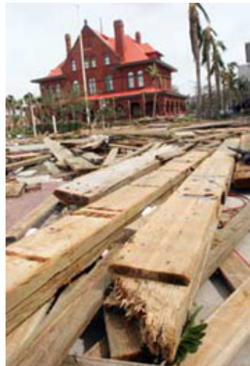
Historic Customs House in Key West, Fla., stands behind remains of Hilton pier torn apart by Hurricane Wilma (photo: Key West Citizen)
